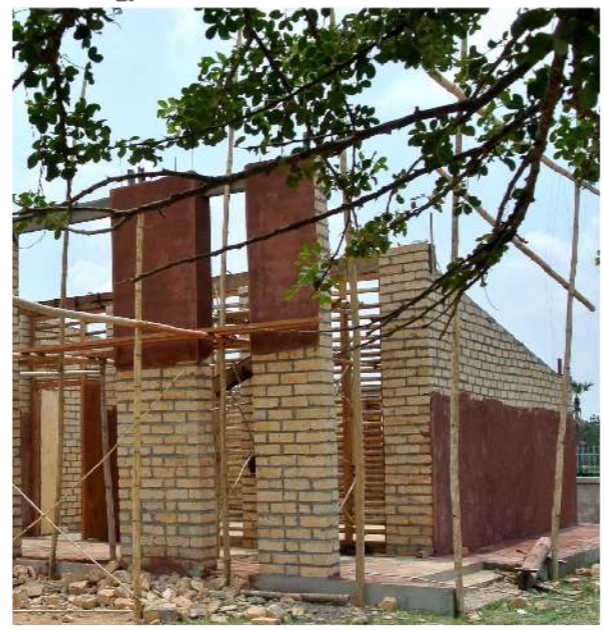
soil block sun-dried with vertical stiffening technology
