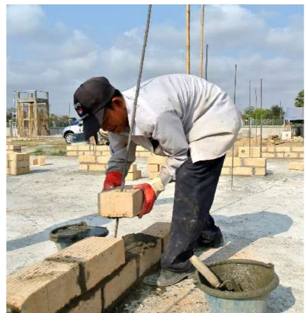
soil block sun-dried with vertical stiffening technology
