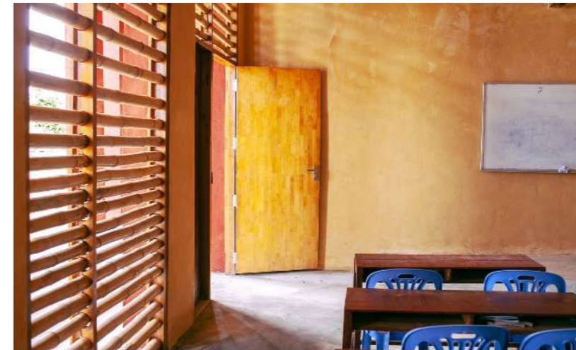
bamboo panels as a separation between hallway and classrooms
