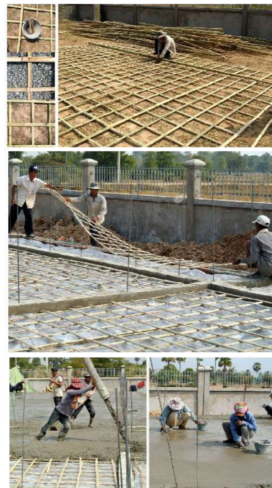
experimental bamboo mesh for the concrete basement
