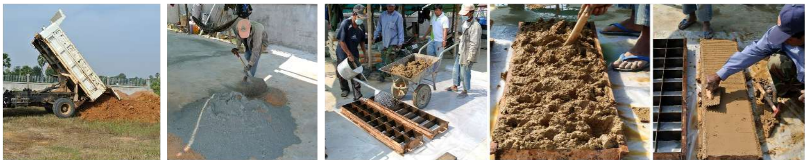
transferable techniques: constructing soil blocks
